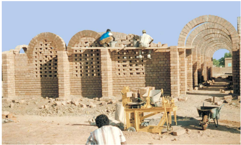
Figure 7.1 - El Haj Yousif school under construction
